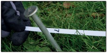
Pull out the measuring tape and put a tent peg by the marking. Use the mounting cross and the measuring tape to position eight tent pegs in a circle.
