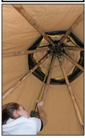
6. Lift the Nordic tipi straight up so that it almost takes on its final shape but don't lift it too high because that will make it difficult to fit in the across-poles.
